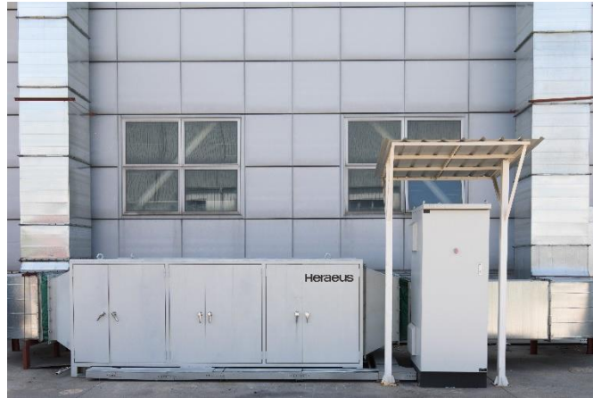
Picture 39: Diagram of Heraeus UV Air Treatment System for Industrial Waste Air
